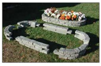
Select a layout configuration; some suggested layouts are on the previous page, or design your own. Lay the RockLock Wall System modules down in the rough locations.
