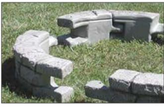
Make sure the rock-textured surfaces of the modules face the outside of the structure, with the rock-textured top surfaces facing up.
