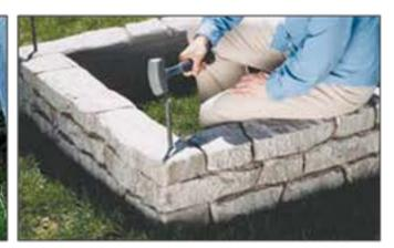
When you are finished, make sure the structure is where you want it to be, then hammer the steel spikes into the ground.
