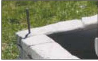
Insert a spike to secure the 2 sections together, but do not hammer into the ground until you are finished with the complete layout.
