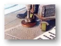
The Safety Grooving Process uses special diamond tools to score shallow grooves into existing floors, decks and walkways. A patented diamond cutting disk is attached to a high speed drill motor which is mounted on to a small weighted cart. A water source is connected to the machine. The water is used to lubricate and cool the diamond bits as it suspends the cutting residue in a liquid slurry.
